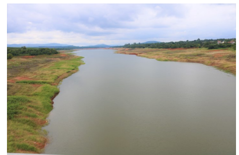
A view of Tzaneen Dam
